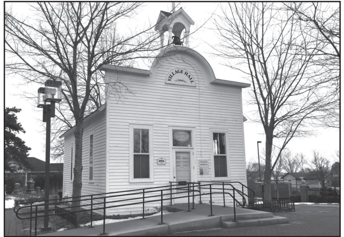
Old Village Hall in Chanhassen
